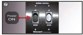
Locate your screen controls and flip the switch to the screen for the deployed position, so that the motor will be receiving AC power.
